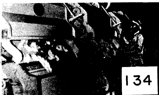
At the Cotton Gin, machines called gin stands pull the cotton fibers off the seeds. Other machines clean the fibers.
