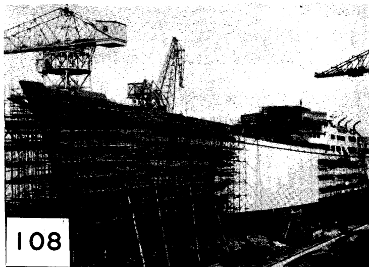
A nearly completed ship stands in the ways, flanked by other partially completed vessels. Many finishing jobs are done in the ways, while others are done after launching.
