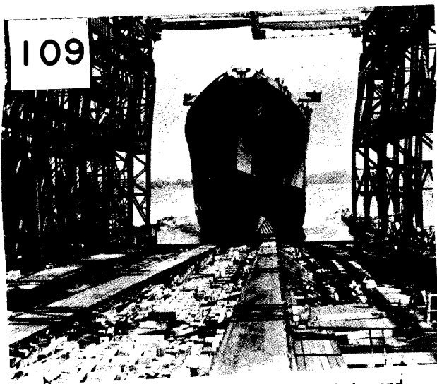
109 A completed vessel runs down the slide ways during end launching, which is accomplished at right angles to the shore line. Side launching is done parallel to the shore.
